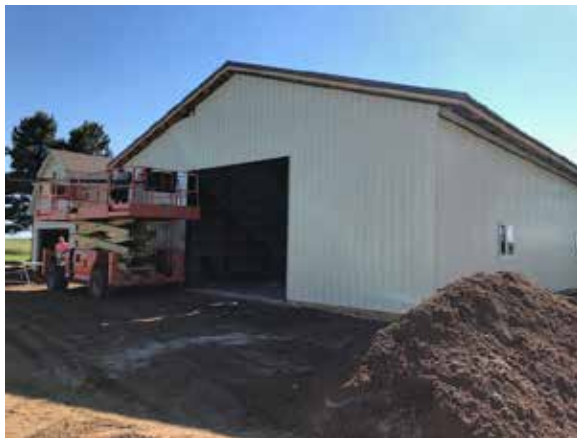
New "Garage" almost complete
